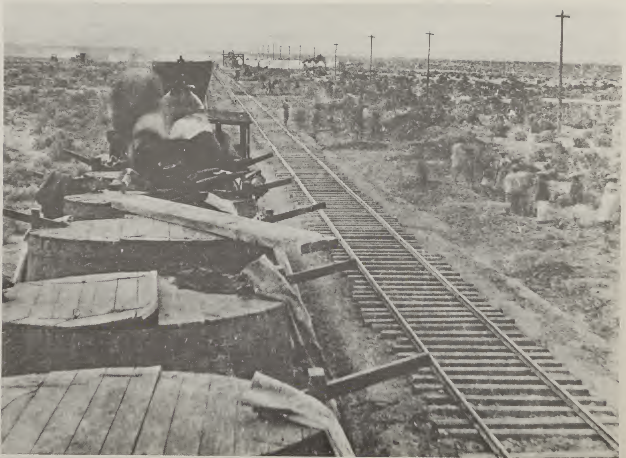
Figure 5: A water train on a siding during construction of the railroad. Note the Chinese laborers to the side of the track (Southern Pacific, Alfred A. Hart Photograph).
